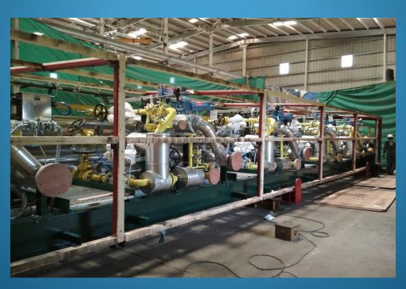
Pressure Swing Adsorber Piping & Valve Skid for Brahmaputra Polymers & Crackers
